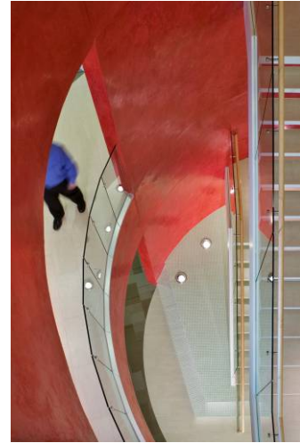
The central stair, with recycled steel and glass surround, transfers light vertically through the 3-level office.
